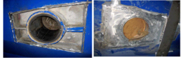
Figure 20: Cutting and welding on the double hull.
