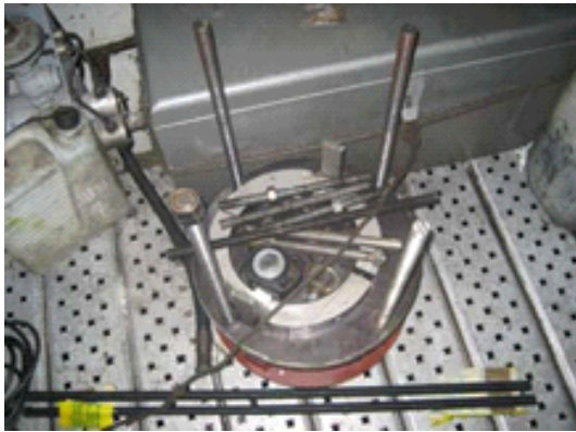
Figure 12: Dismantling of the bearing system of the Roll-fin.
