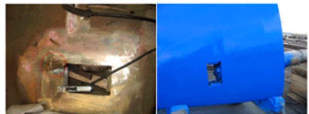
Figure 17: Repair of the crack and painting of the rudder.
