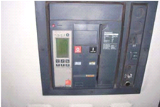
Figure 11: Motorised circuit breaker with an electronic control of 690V.
