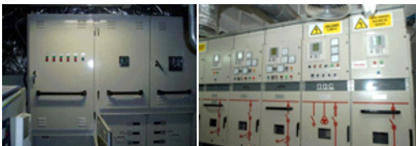
Figure 8: Distribution Boards of the Trimaran and the Methane Vessel.
