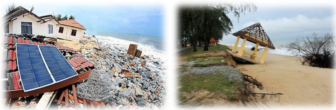
Figure 1: Destroyed existing breakwaters and facilities near to the beach.
