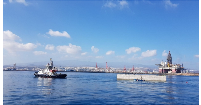
Figure 11: Tugboat towing a box for its final positioning.
