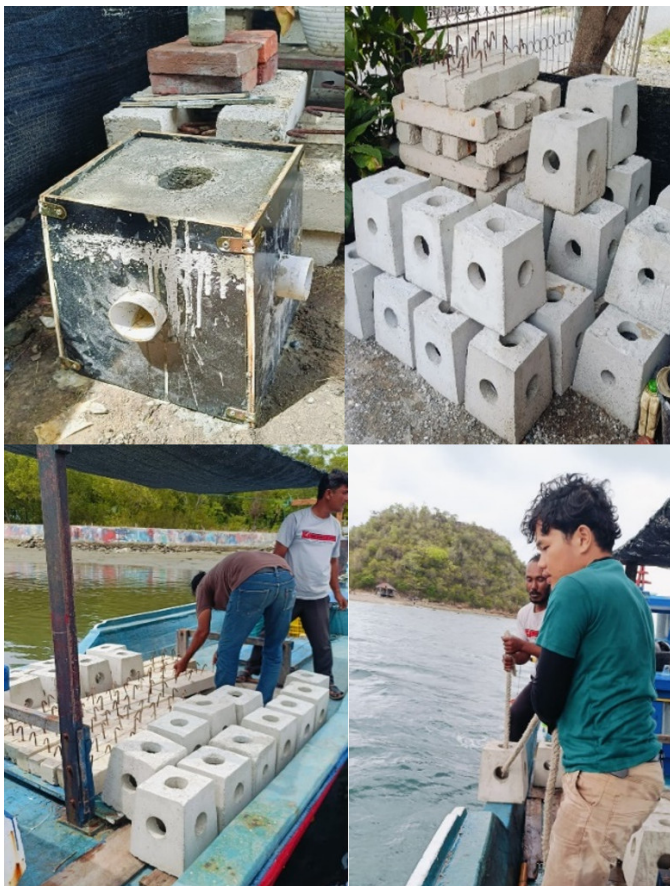
Figure 5: The structure is made and placed under water.
