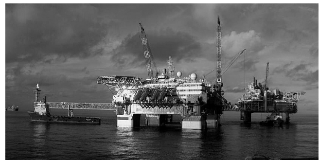
Figure 1: Floatel Superior Semi-Submersible Offshore Flotel on Bayo Undan Oil Field
