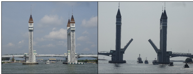
Figure 1: Kuala Terengganu Drawbridge (KTD) closed (left) and open (right).
