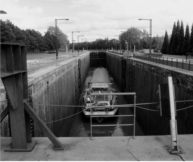
Figure 3: A ship inside the downstream lock (Fontinettes) during the filling process.
