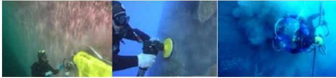
Figure 4: Traditional Underwater Hull Cleaning Methods.
